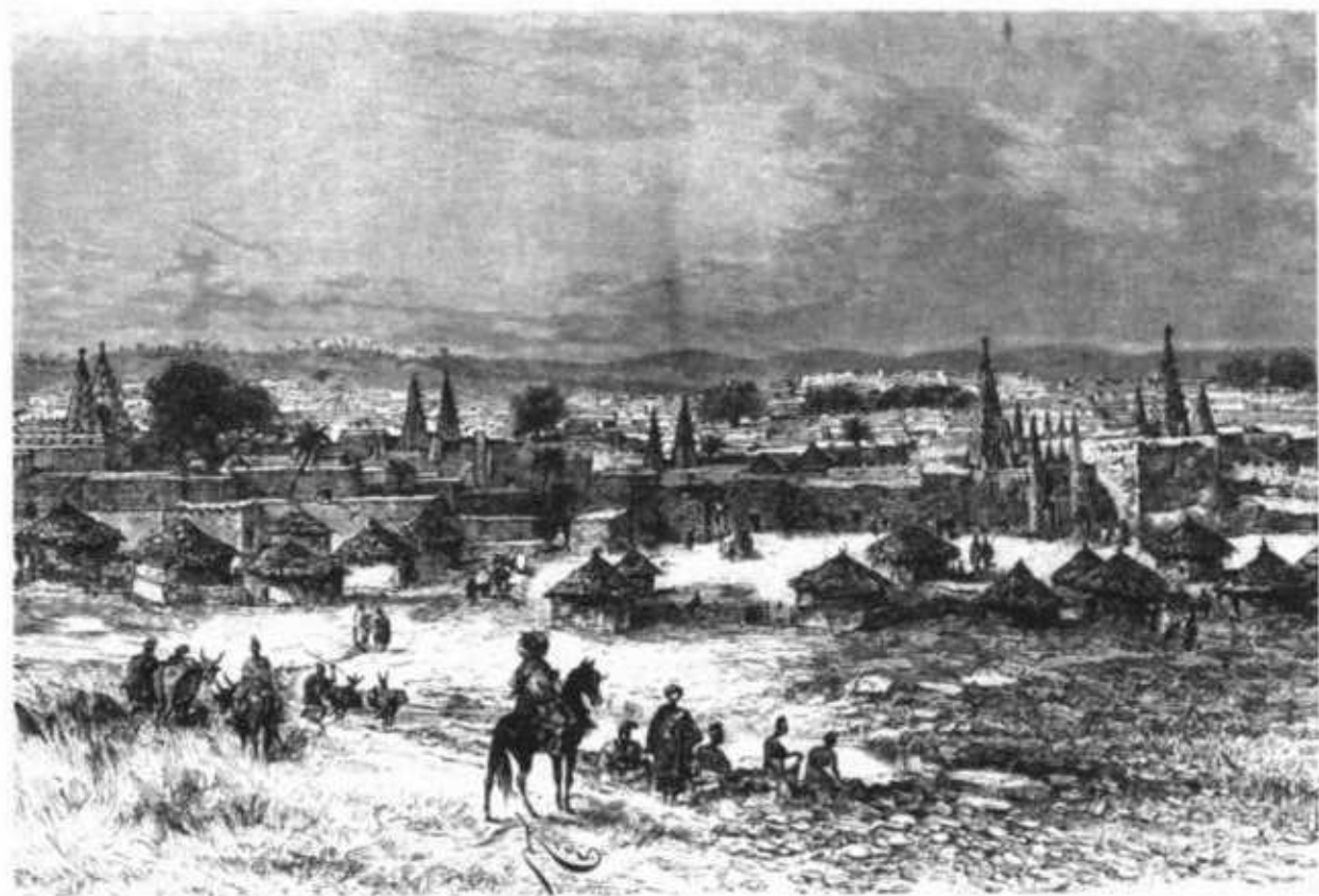
PLATE 12.3 General view of Kong
