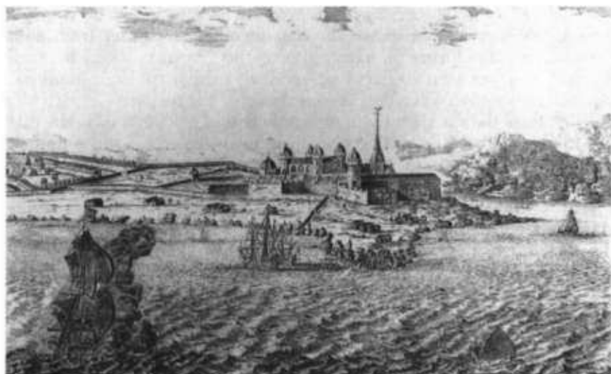
PLATE 14.1 Fort St George at El Mina, as it was in the time of the Portuguese
